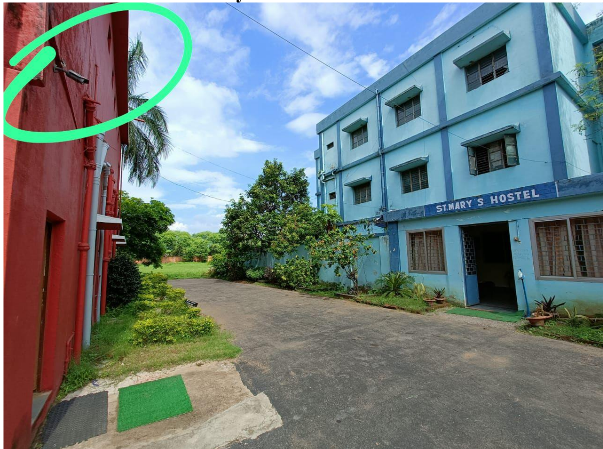
CCTV in front of St. Mary's Girls Hostel
